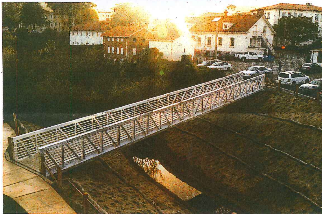
A basic 95-foot-long footbridge in Tennessee Hollow was meant to be simple and affordable.
