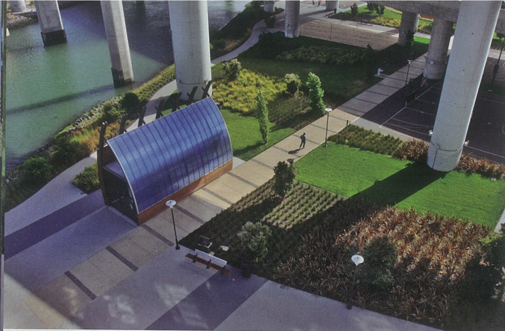
LEFT: A rich and colorful landscape weaves in and out of Mission Creek Park North expressing wave like patterns and a playful reflection of the sculptural ramps above. Dynamic and colorful during the daytime and nighttime, the kayak storage building coveys more of the park's nautical and playful theme. PHOTO COURTESY OF MARCIA LIEBERMAN
