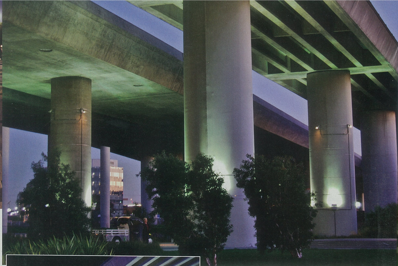
ABOVE: Strangely akin to a forest of large sequoia trees, these large concrete supports (called bents) and their accompanying freeway ramps create a unique spatial environment for pedestrians in this active sports park. Reflected light from the indirectly illuminated freeway canopy helps to softly illuminate large areas of the park that otherwise do not have any specific pole lighting nearby.
