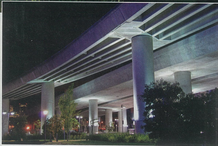
ABOVE: Strangely akin to a forest of large sequoia trees, these large concrete supports (called bents) and their accompanying freeway ramps create a unique spatial environment for pedestrians in this active sports park. Reflected light from the indirectly illuminated freeway canopy helps to softly illuminate large areas of the park that otherwise do not have any specific pole lighting nearby.
