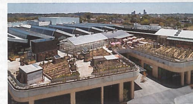
THE BULLITT CENTER , in Seattle (top), and the Kendeda Building, in Atlanta (middle), both by Miller Hull, meet the LBC net-positive energy requirement with expansive PV arrays. A shopping mall (bottom) in Melbourne, pursuing certification, has a rooftop farm.
